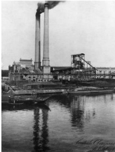
Fig.1 The power plant Oberspree was built outside the city centre in 1896/97. It had its own harbour to improve the supply with coal. It is one of the oldest three-phase power plants in Europe and still preserved. (Source: Vattenfall Europe, Historical Archives, Berlin)
